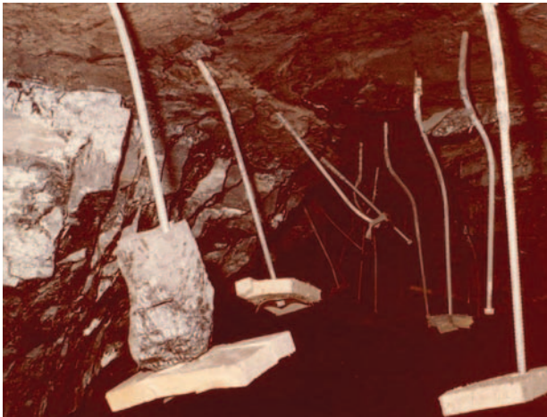
Figure 5. Typical roof fall caused by excessive pillar loads.
