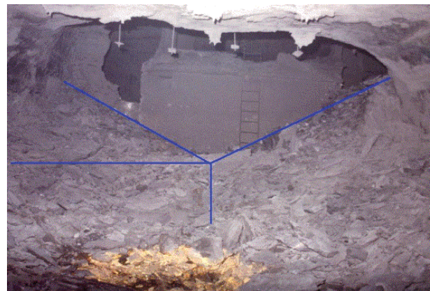
Figure 3. A scaled pillar indicating the angle of repose and the height of the rubble (after Canbulat and Ryder, 2002).
