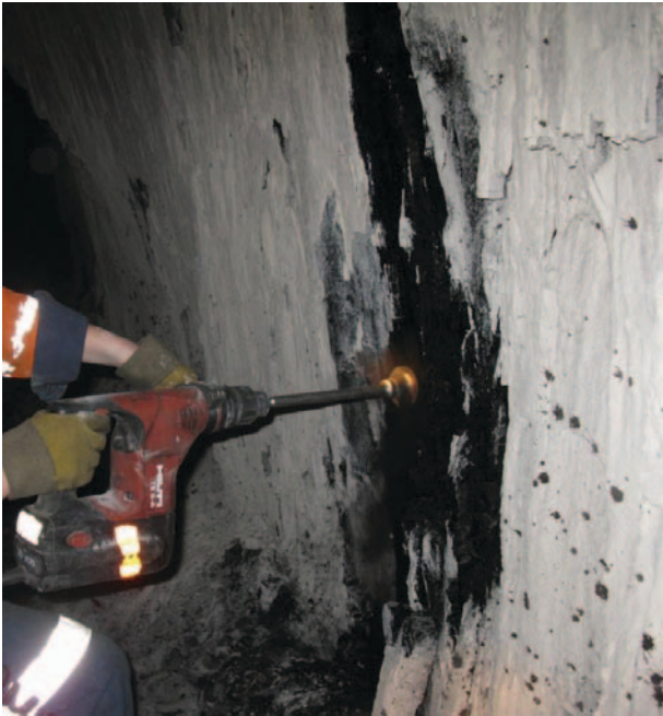
Figure 4. Coring using the Hilti portable drill.
