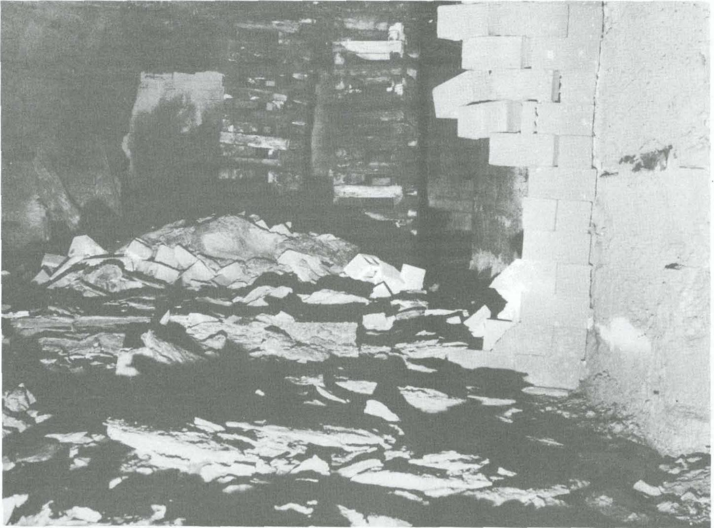
Figure 2. Concrete cinder block stopping damaged by airblast.
