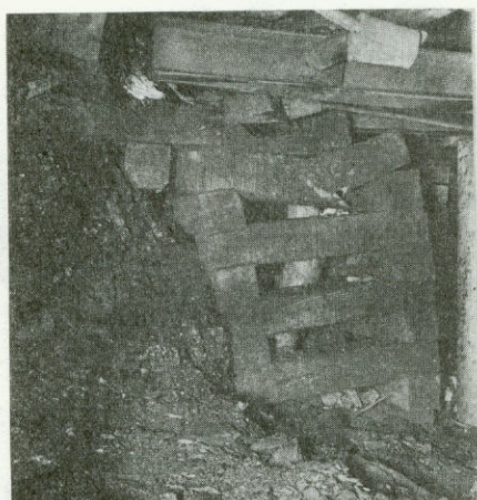
(c) 1st Stage Deformation of Ribside/Cog - 2nd Face Extraction
