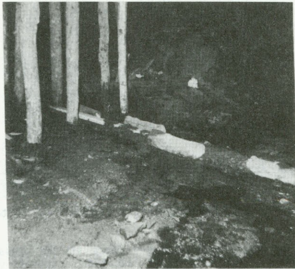
Picture 3 Protection of Pressure Lines by 5 \times 10 cm ( 2 \times 4 in.) Timbers, End Pieces of Posts and Dirt
