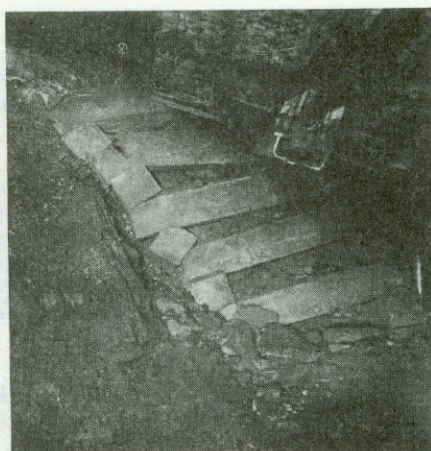
(d) 2nd Stage Deformation of Ribside/Cog - 2nd Face Extraction
