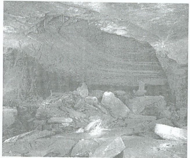
Figure 4. - If the roof is not reinforced properly with rock bolts, the beams can progressively fail higher into the roof until a stable roof beam is encountered. Here the roof fall has assumed an elliptical shape.
