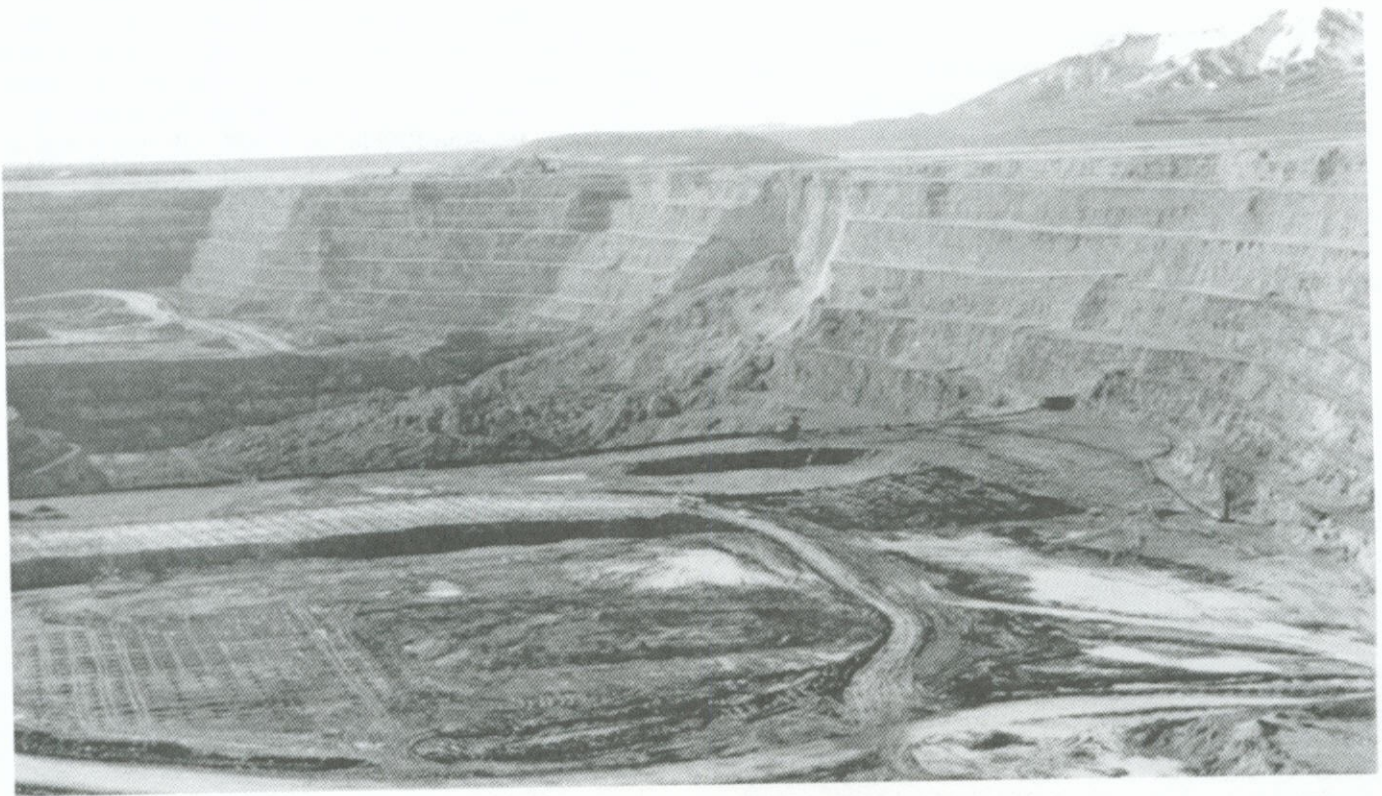
Figure 1 -- Massive slope failure in the highwall of an open pit mine.
