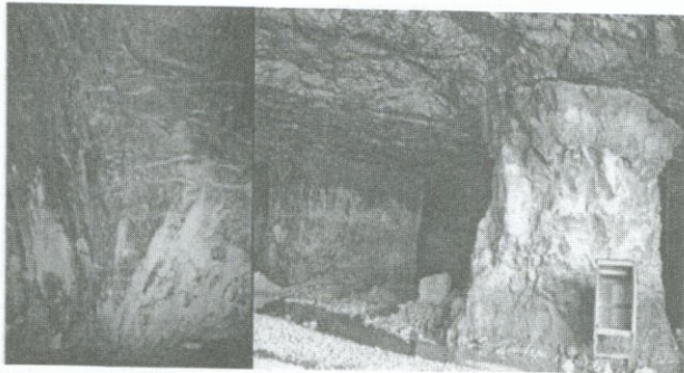
Figure 1 - Photographs of failing pillars. Photo on left shows a crushed edge with a concaved shape and photo on right shows a failed pillar in the foreground [Note the crushed ribs and the slender appearance, w/h < 1 while the pillar in the background is stable with a w/h > 1 ].
