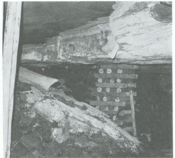
Figure 7 In general the roof was in good condition, although some falls of 0,5 to 1 m had occurred.
