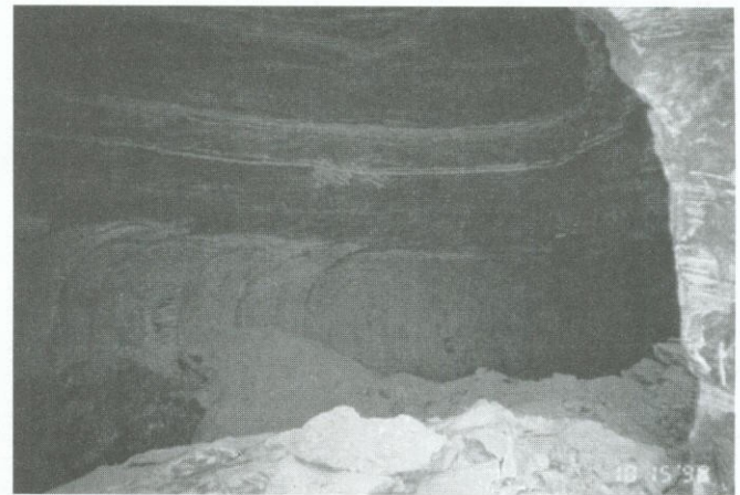
Figure 6b. View of Dome-shaped Roof Fall from Crosscut
