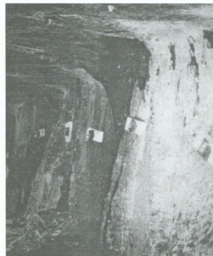
Figure 4. Skin failure of supported rib.
