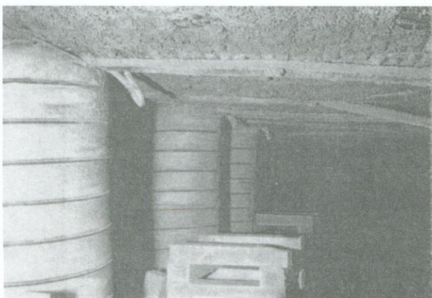
Figure 11a. Outby area supported with pumpable crib.
