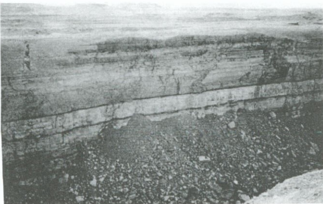
Figure 2 - Failed highwall slope resulting from sudden web pillar collapse.
