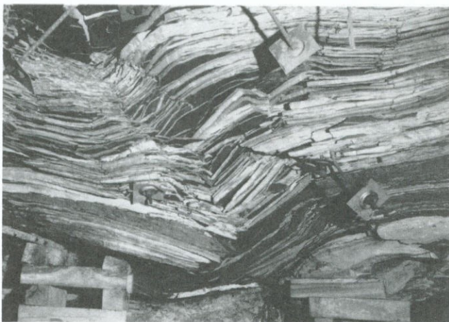
Figure 3. Cutter roof failure.
