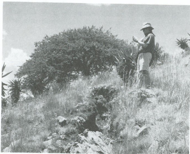
Figure 13 Part of the fresh crack that was found, associated with the Alfred seam collapse.
