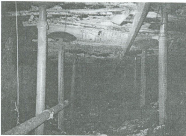
Figure 13b. Inby area supported by ACS supports.
