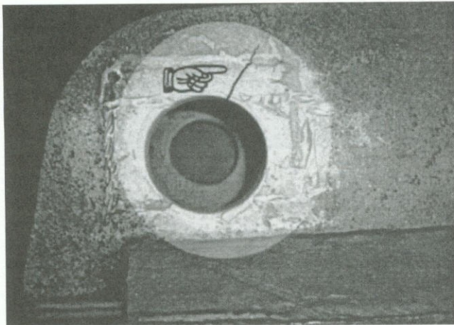
Figure 13. Failure in base lemniscate link clevis.
