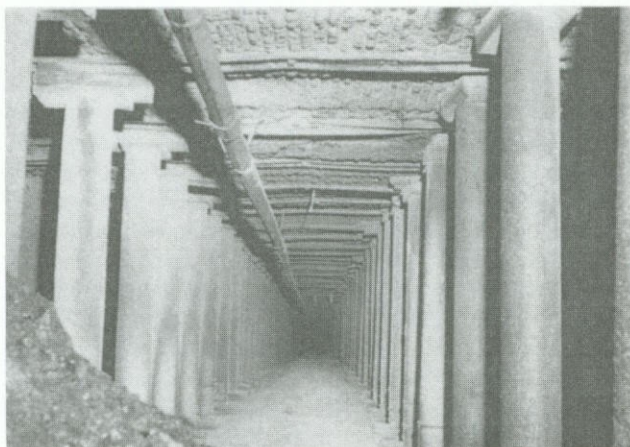
Figure 12a. Outby area supported by Propsetter support.
