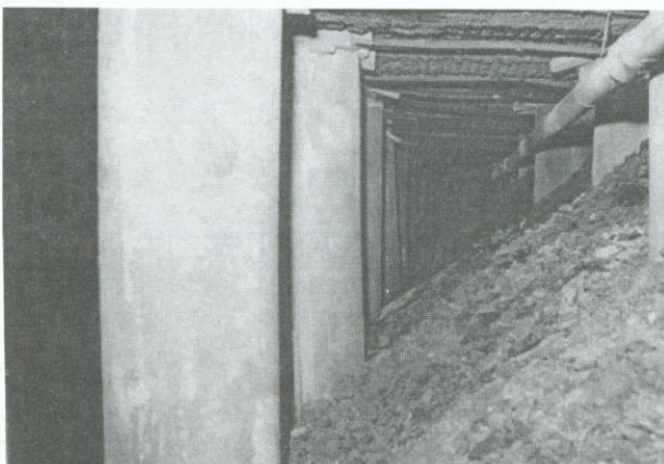
Figure 14b. Inby area supported by the Can Support.
