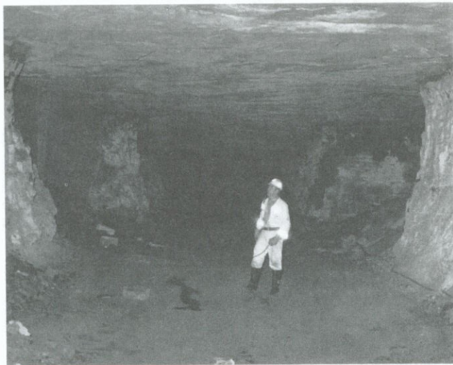
Figure 5 The workings in the area where the pillars did not collapse was about 4 m high.
