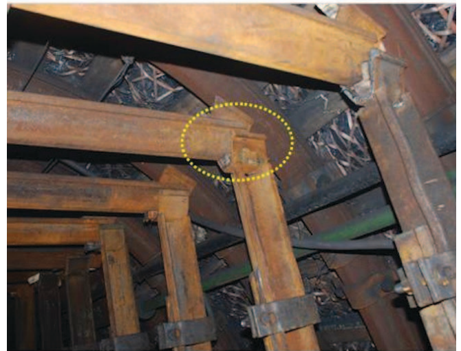
Figure 17. Connecting parts of the U-steel support.
