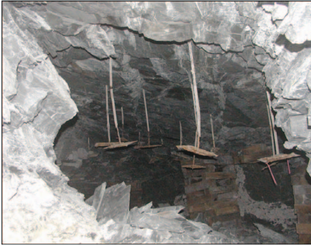
Figure 16. An example of coal mine shale roof unraveling between roof bolts in response to internal strains and reduction in rock strength caused by moisture adsorption.
