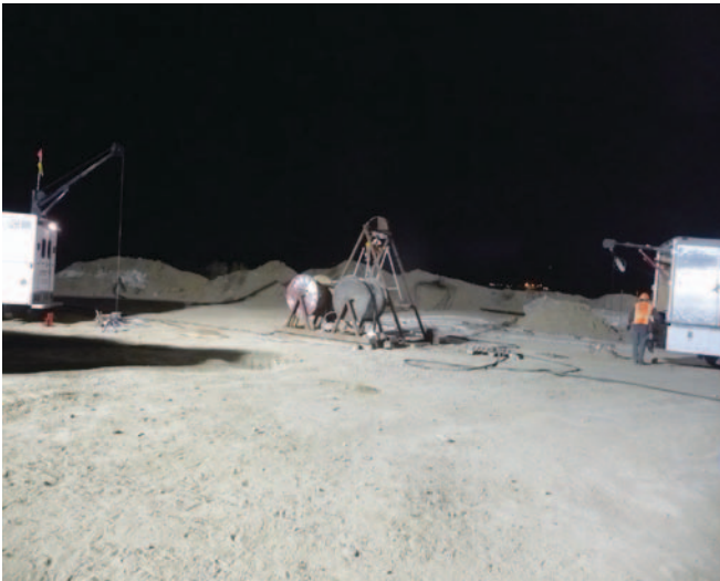
Figure 8. Pumping from surface.
