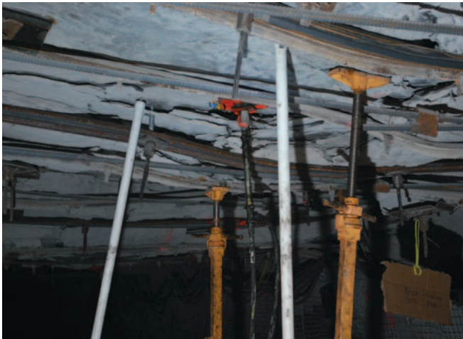
Figure 5. Polyurethane injection for strata consolidation.
