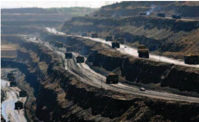
Figure 2. Haulage road in the end-walls.
