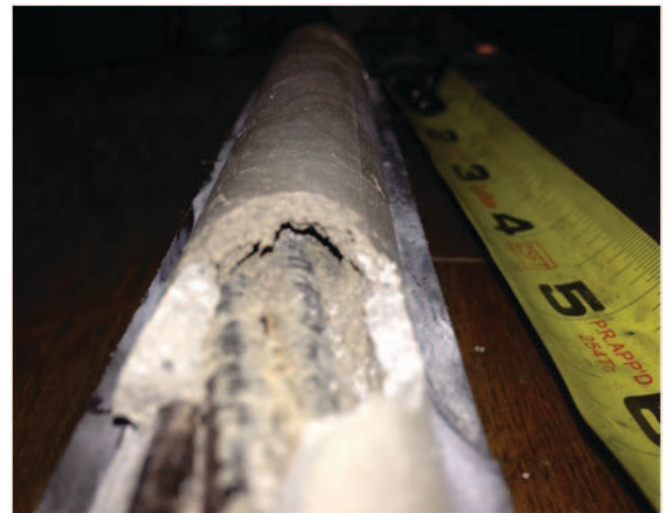
Figure 8. Void detected in sectioned bore tube sample of indented cable with counter clockwise rotation.
