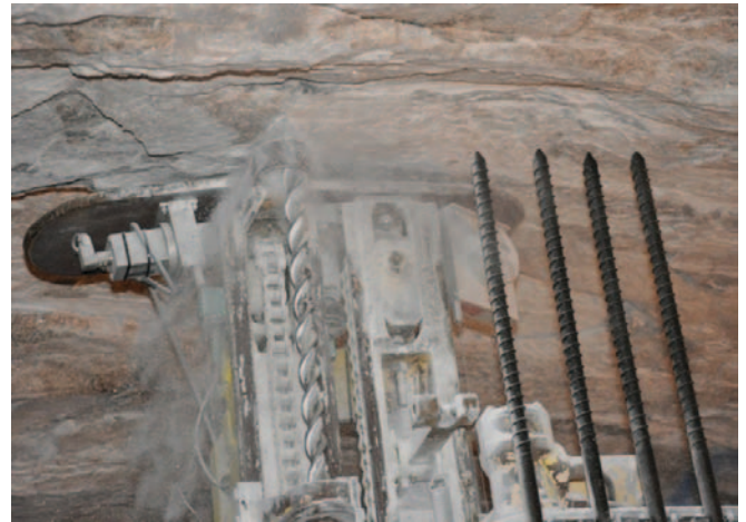
Figure 8. Stepped drill bit in operation.
