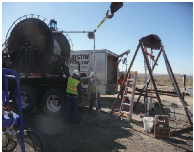
Figure 7. Lowering hoses from surface.
