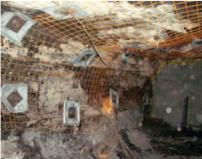
Figure 5. Example of the additional rib support systems used throughout the take-off areas.
