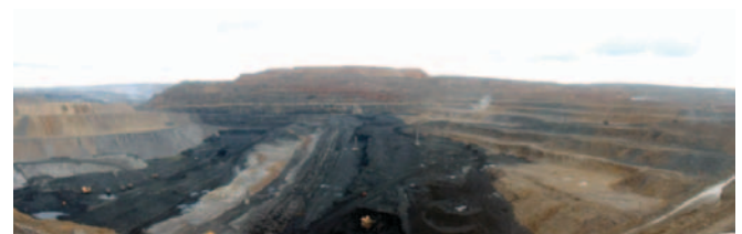
Figure 4. Working pit and end-wall at AKB coal mine, China.
