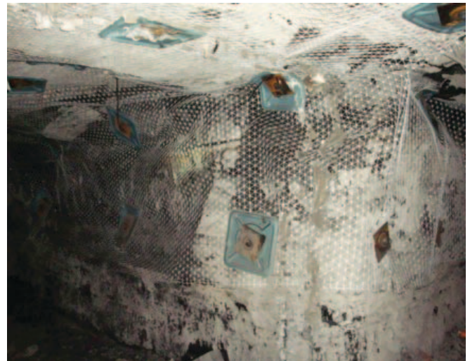
Figure 6. The completed roof and rib support systems.
