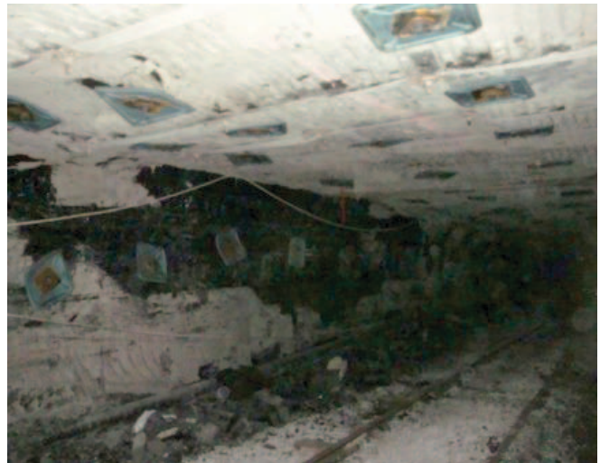
Figure 4. The supported longwall entry after additional supports were installed.
