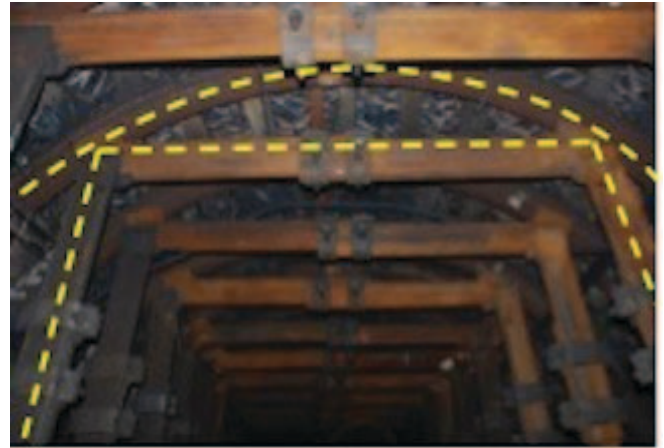
Figure 16. Structurally enhanced U36 steel support.
